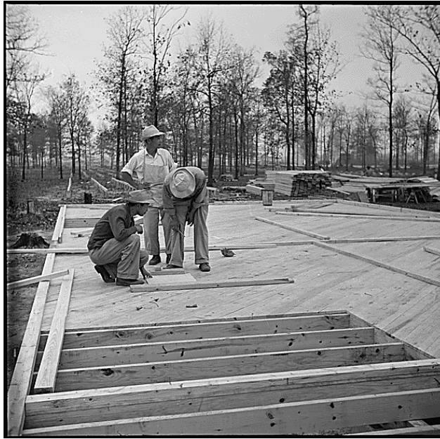
Photograph NO. NWDNS-210G-E308. Rohwer Relocation Center, McGehee, Arkansas. Volunteer workers are here constructing apartments for the administrative staff. National Archives and Records Administration. Photographer: Tom Parker
